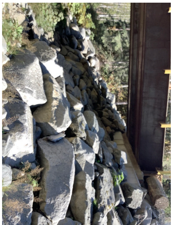
Right Bank Abutment when facing downstream
